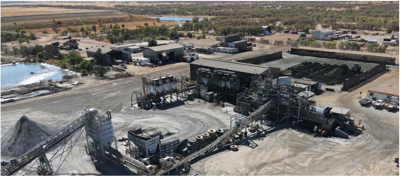
Eloise Copper Mill – Credits AIC Mines
