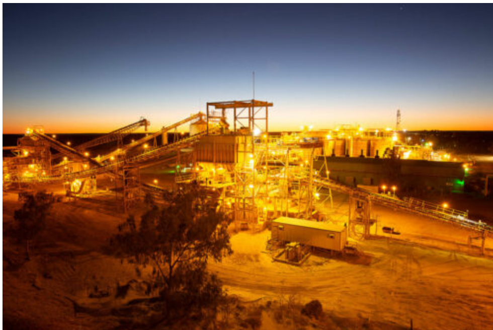
Plutonic Gold Mine at night – Courtesy of Catalyst Metals Ltd.
