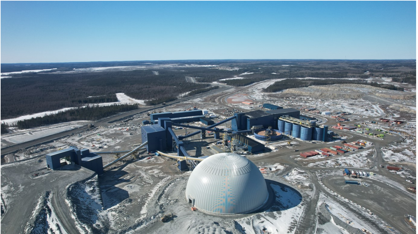
Greenstone Mine – Credits Equinox Gold Corp.
