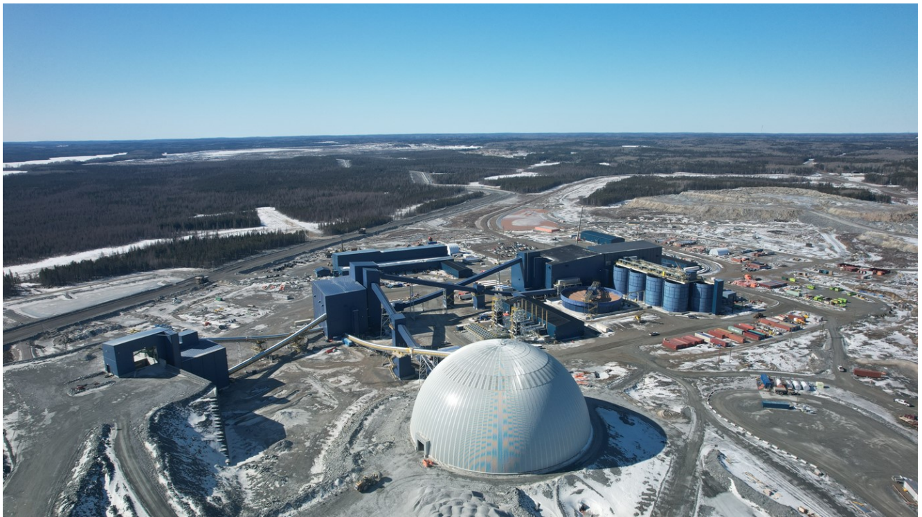
Greenstone Mine – Credits Equinox Gold Corp.
