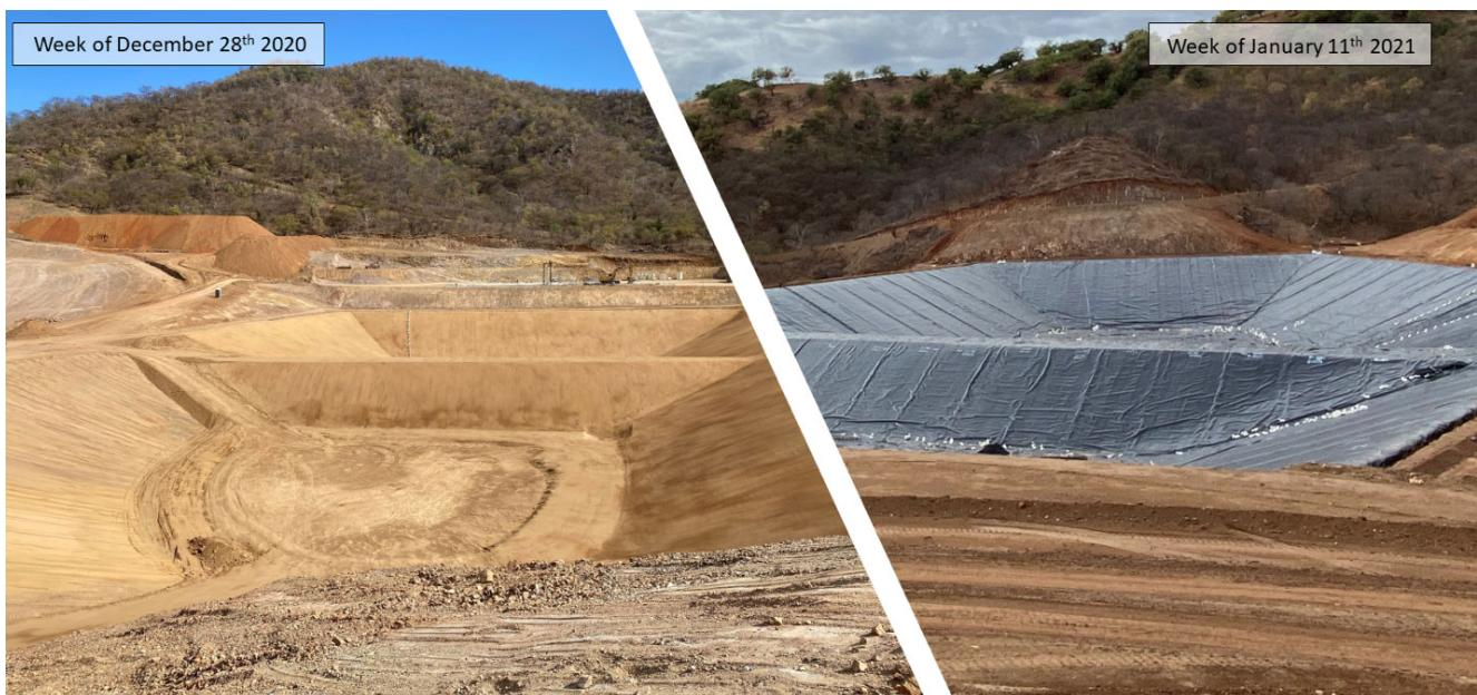
With the vast amount of construction activity in 2020 revolving around earthworks for the plant, ponds and pad the final installation of liners and plant process equipment is moving forward quite rapidly as can be seen in the transition from unlined to fully lined ponds in just a few weeks (Photo 1). The main pad liner is expected to be installed over the coming weeks in parallel with the final installation and connection of equipment related to the gold recovery plant.
