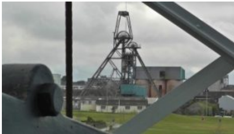
South Crofty Mine headframe, near Cambourne, Cornwall, England.
