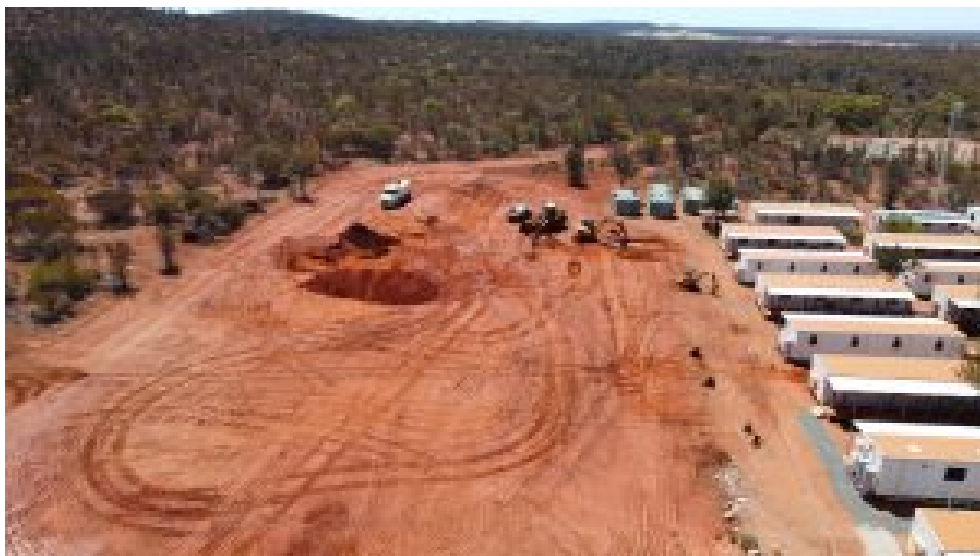
Site View – Courtesy of Ora Banda Mining
