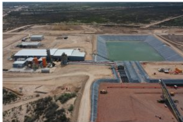
Orla Mining heap leach pad, Solution pond, and Merrill-Crowe plant – Credit Orla Mining
