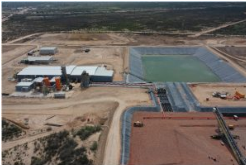
Heap leach pad, Solution pond, and Merrill-Crowe plant – Credits Orla Mining
