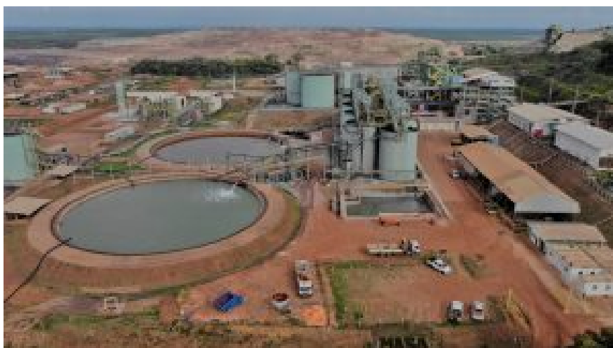
Aurizona Mine, Brazil – Credit Equinox Gold
