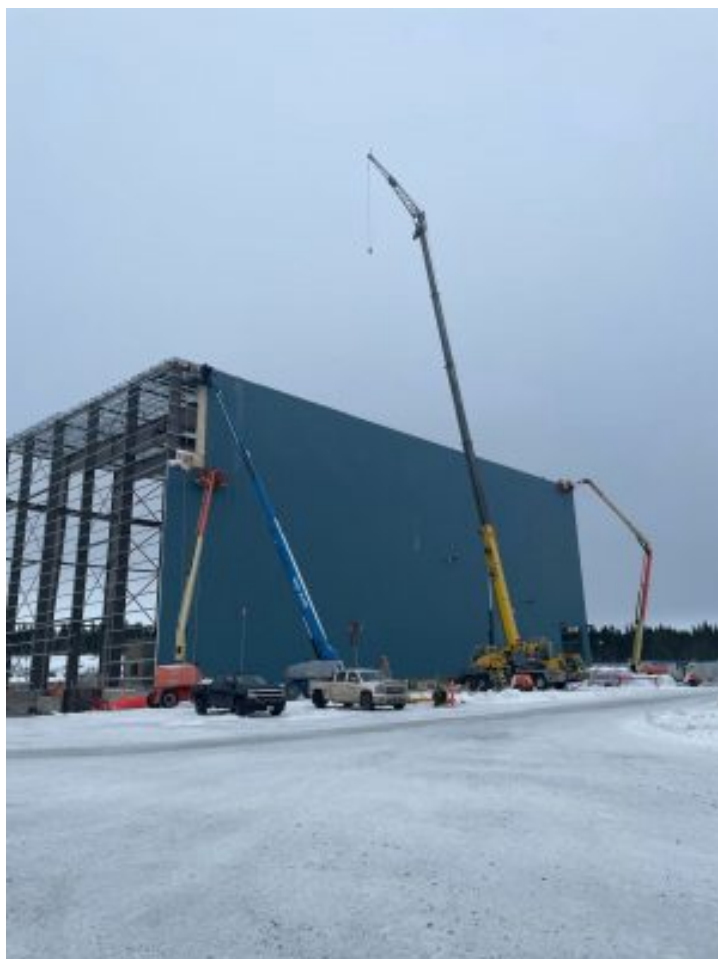
Calibre Mining Valentine mine construction
