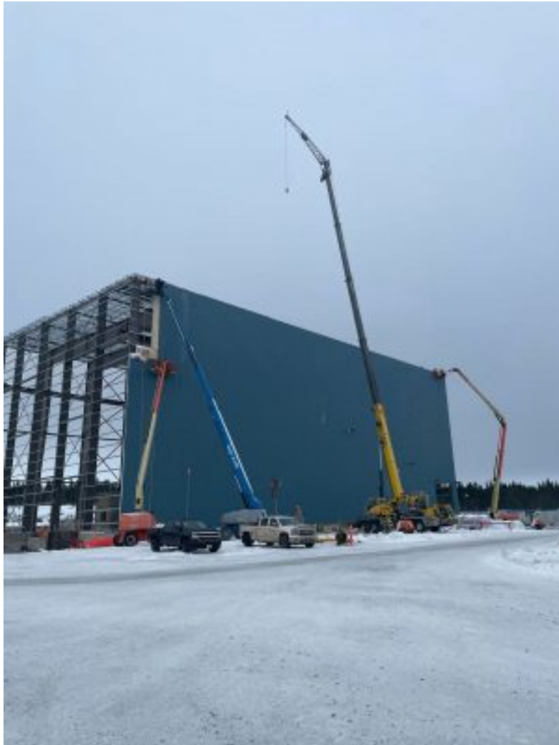
Calibre Mining Valentine mine construction
