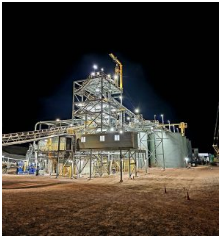
Calidus Resources Warrawoona Mine Plant, WA
