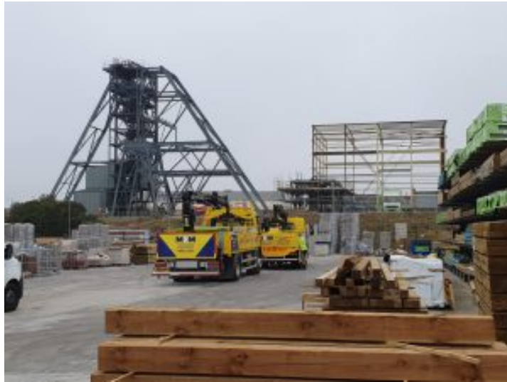
Cornish Metals South Crofty headframe as seen from the adjoining builders merchants yard.
