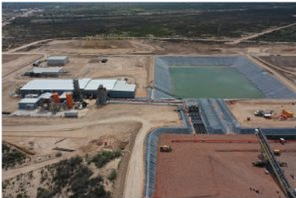
Orla Mining heap leach pad, Solution pond, and Merrill-Crowe plant – Credits Orla Mining Ltd.
