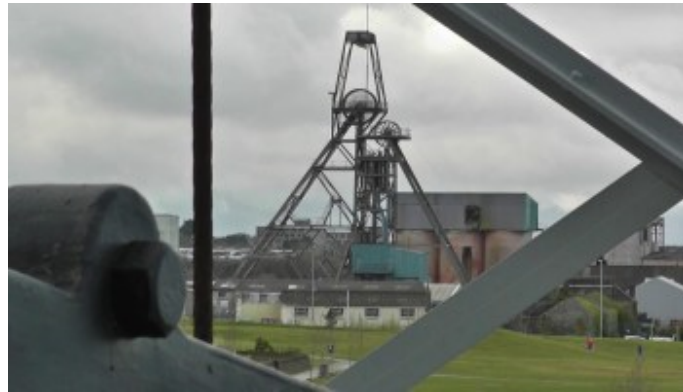
Cornish Metals South Crofty Mine Headframe
