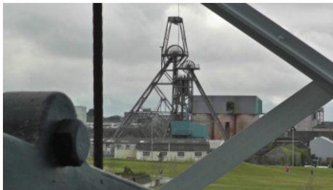
Cornish Metals South Crofty mine, Cornwall, England.
