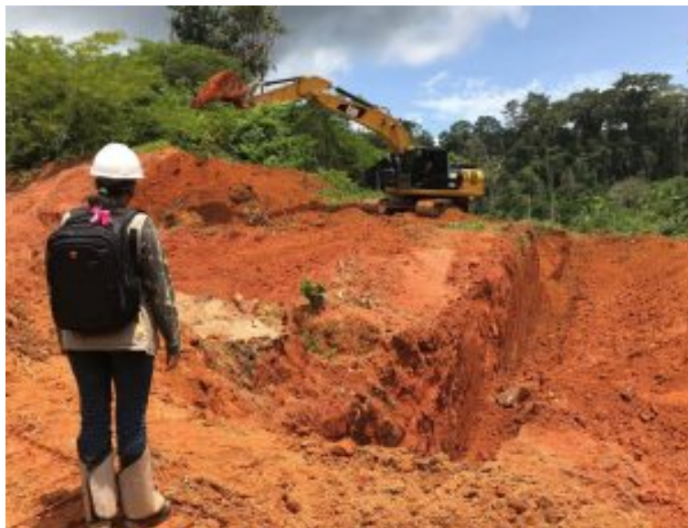
Cuiú Cuiú excavation – Courtesy of Cabral Gold
