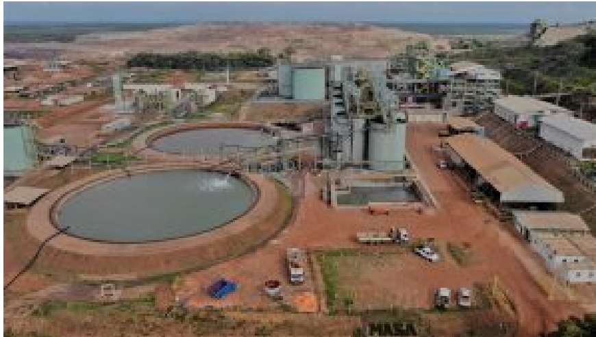
Aurizona Mine, Brazil – Credit Equinox Gold
