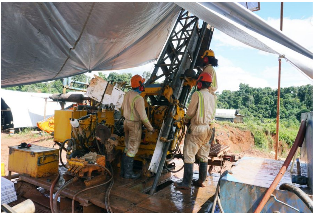
Drilling – Photo courtesy of g2 Goldfields
