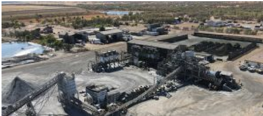
Eloise Copper Mill – Credits AIC Mines
