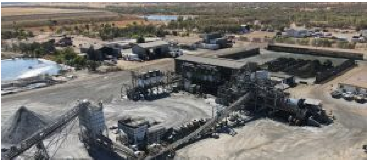
Eloise Copper Mill – Credits AIC Mines
