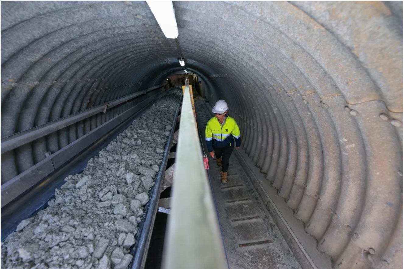
Maldon processing plant – Credits Kaiser Reef Ltd.
