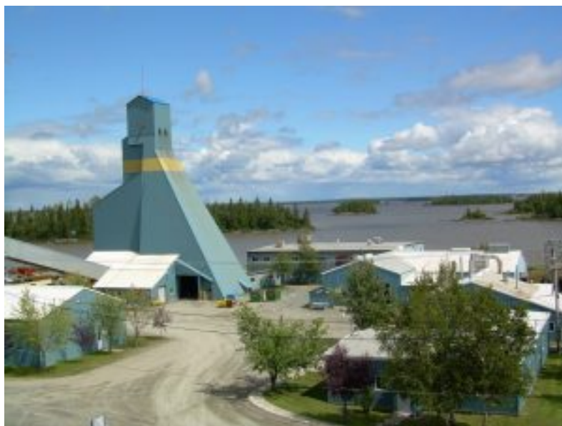
Wesdome Gold Mines Kiena Mine, Quebec
