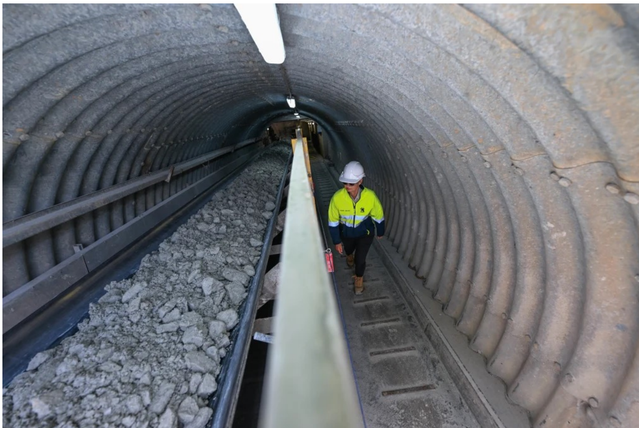
Maldon processing plant – Credits Kaiser Reef Ltd.
