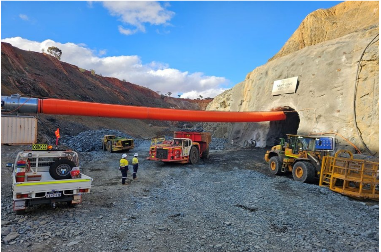
Riverina adit – Courtesy of Ora Banda Mining
