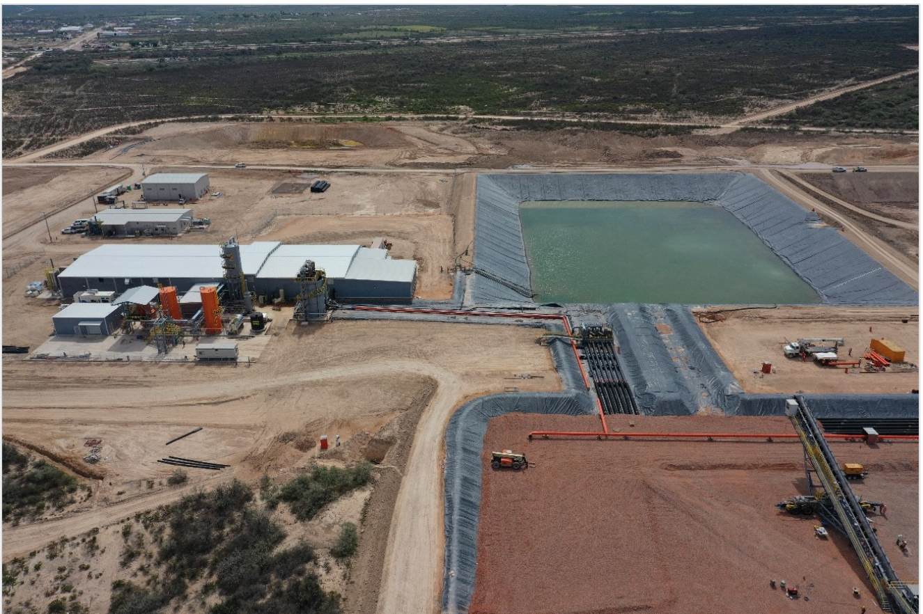
Orla Mining heap leach pad, Solution pond, and Merrill-Crowe plant – Credits Orla Mining
