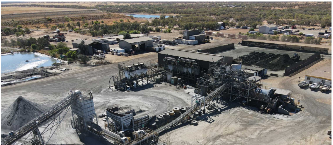
Eloise Copper Mill – Credits AIC Mines
