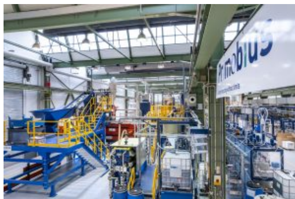
Primobius Werkstatt Hilchenbach Plant, Germany
