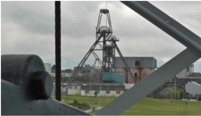
Cornish Metals South Crofty Mine Headframe
