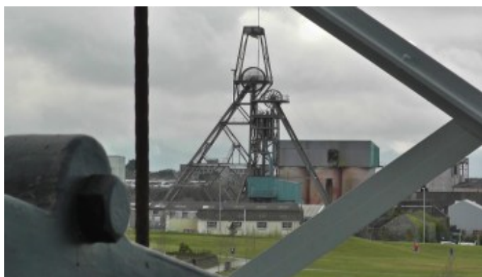
Cornish Metals South Crofty mine, Cornwall, England.
