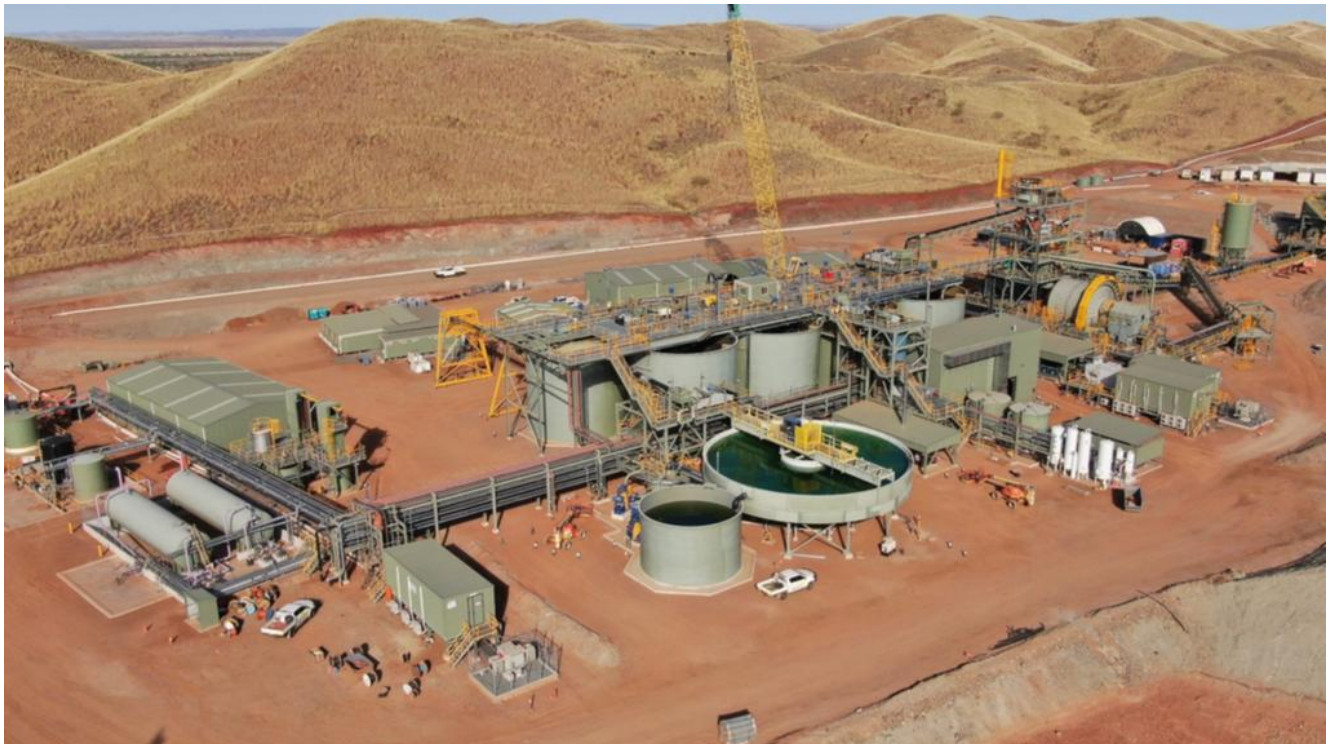
Calidus Resources Warrawoona mine, Pilbarra, Western Australia.
