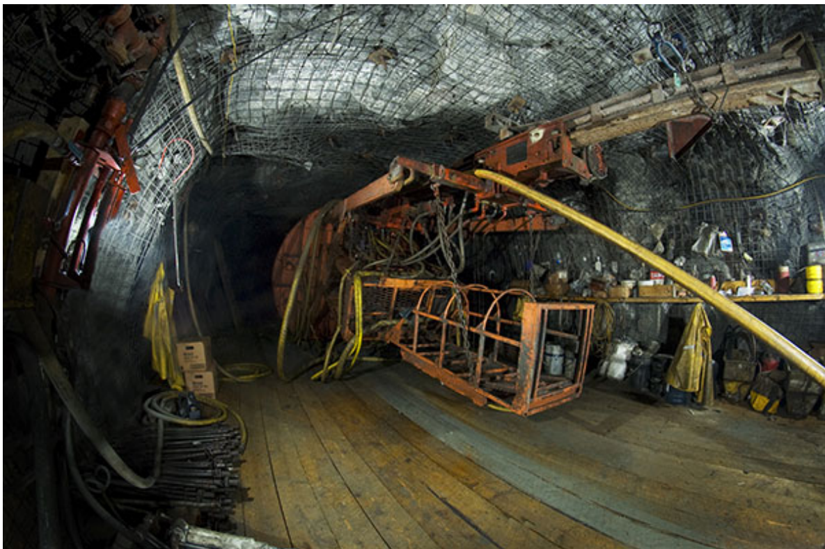
Wesdome Gold Mines – Eagle River underground mine
