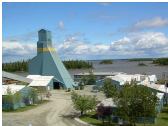
Wesdome Gold Mines Kiena Mine, Quebec
