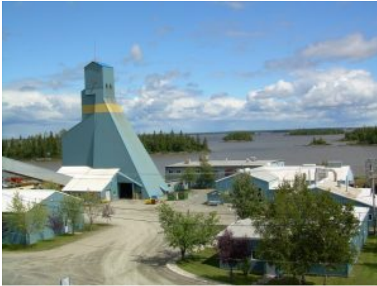
Wesdome Gold Mines Kiena Mine, Quebec.
