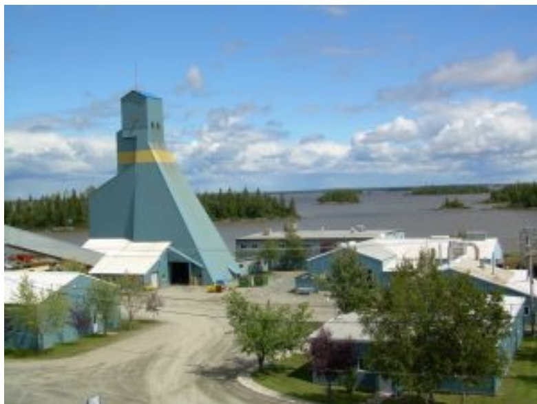
Wesdome Gold Mines Kiena Mine, Quebec
