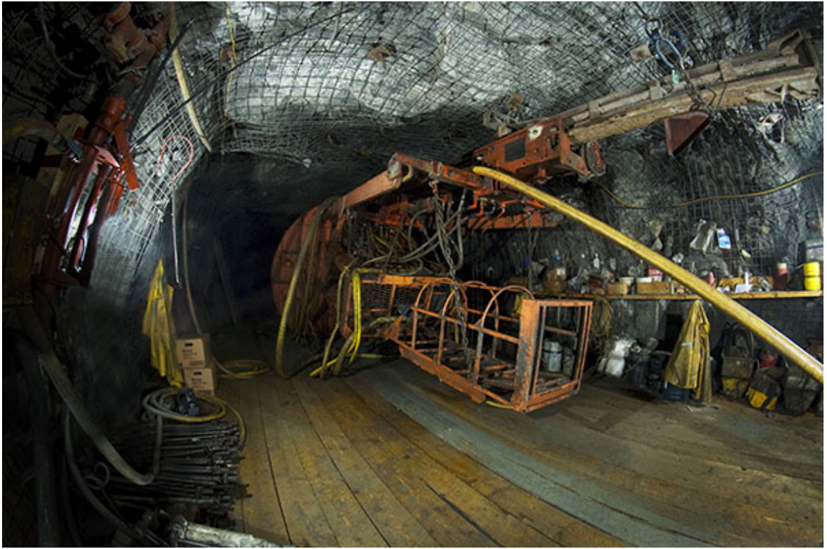
Wesdome Gold Mines – Eagle River underground mine
