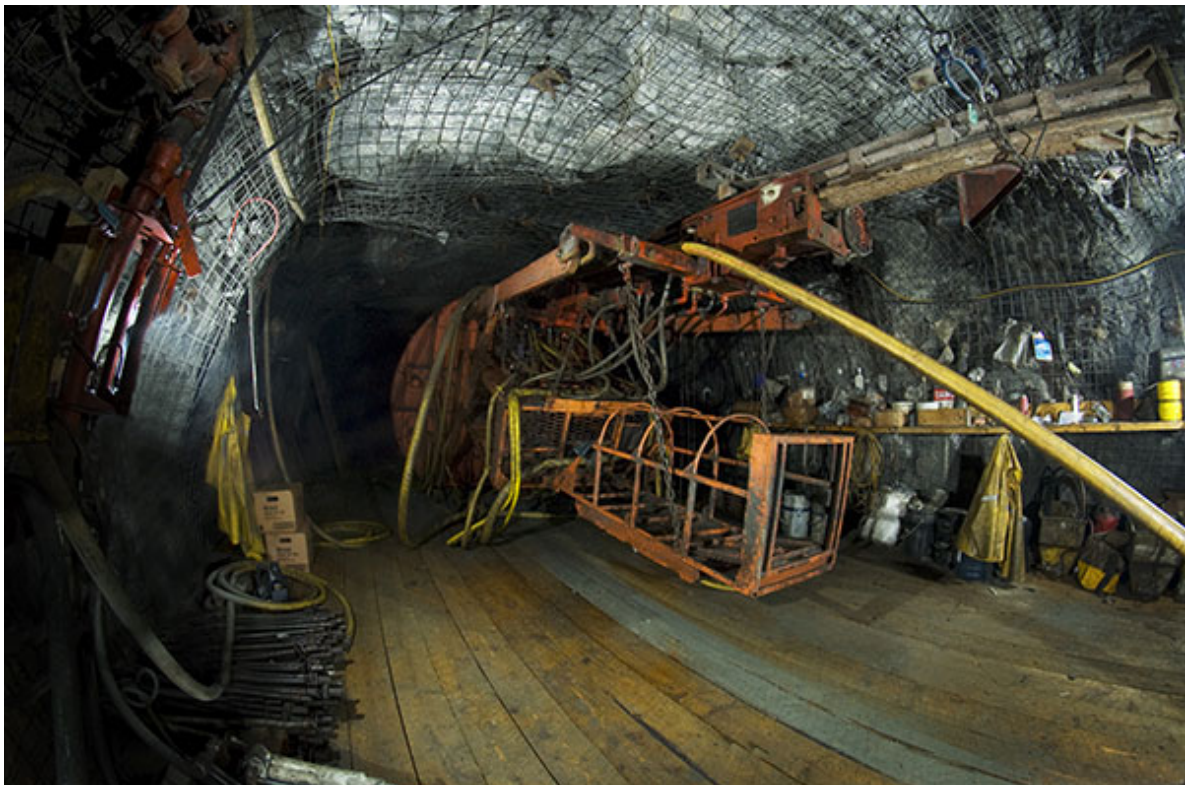
Wesdome Gold Mines – Eagle River underground mine
