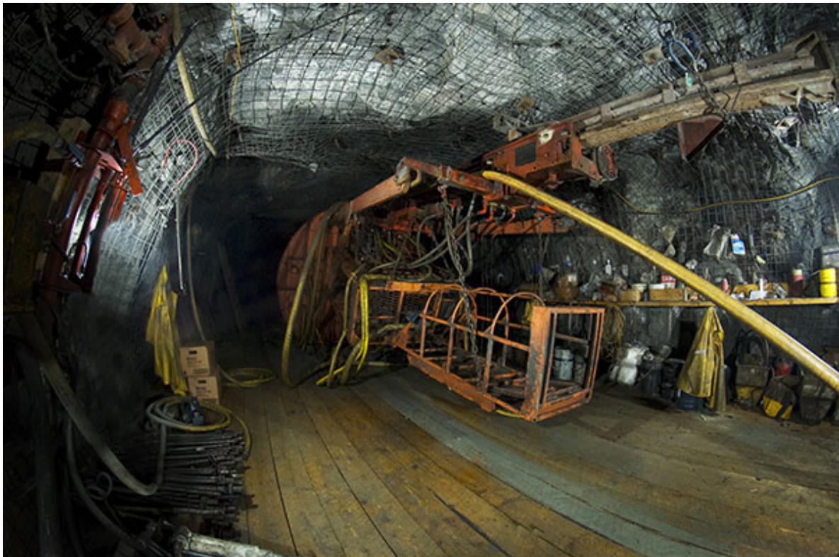
Wesdome Gold Mines – Eagle River underground mine
