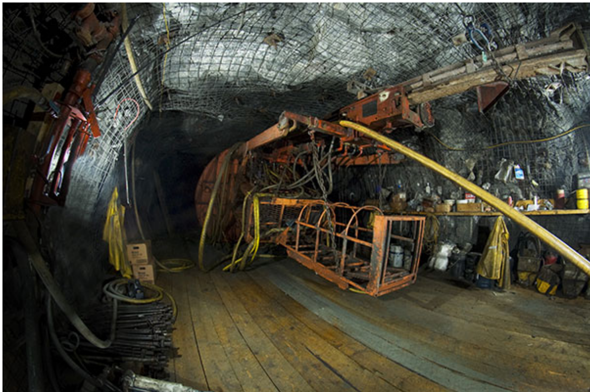
Eagle River underground mine – Courtesy of Wesdome Gold Mines
