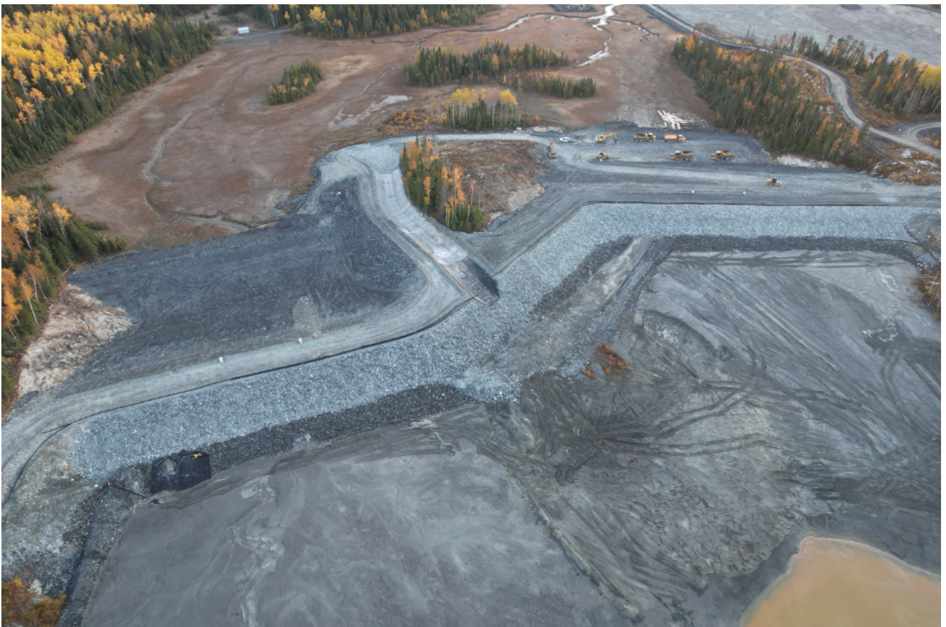
Aerial view of the tailings dam lift project at completion.
